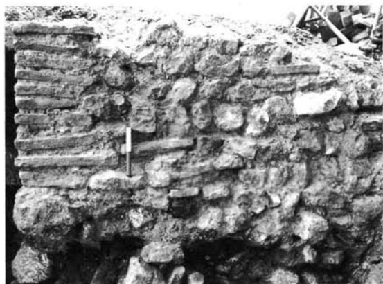
Fig 17. St Olave Jewry (96): details of Roman tiles reused as quoins. Scale is 2 × 100mm units
